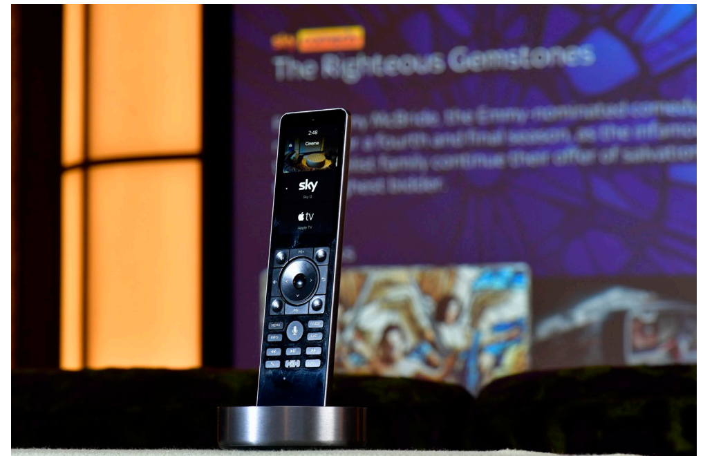
A Savant Pro control system makes the cinema room easy to use
