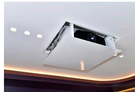
A motorised lift hides the projector in the ceiling when not in use—with lighting either side for the pool table
