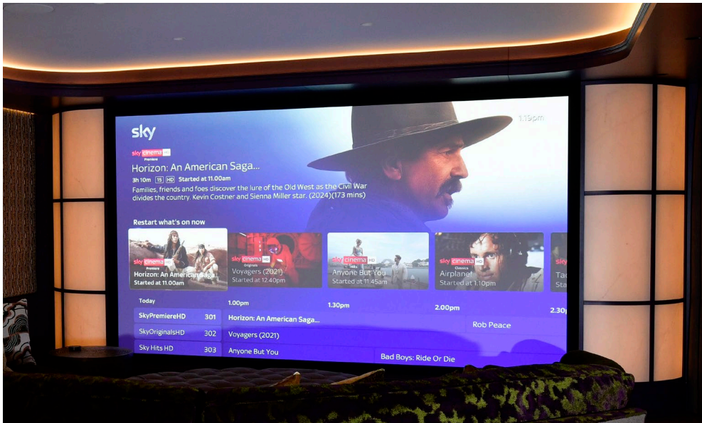
Curved lightboxes were fabricated for either side of the screen to allow space for the LCR (Left, Centre, Right) speakers behind without obscuring the windows
