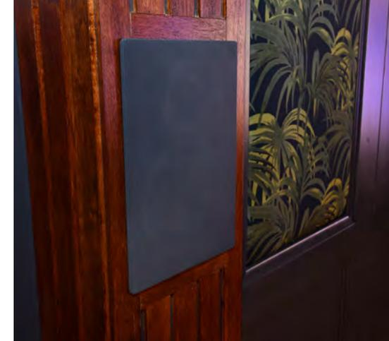
Also hidden at the front are two JL Audio subwoofers that feature an ultra slim outer casing, helping with placement while still providing very large sound pressure levels.
