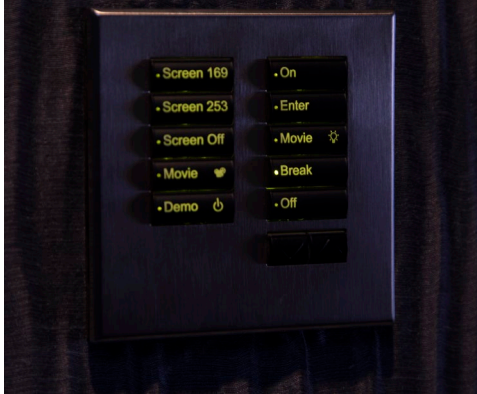
Lutron wallplate allows quick access to main cinema controls.
