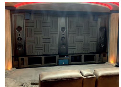
The correct positioning of the Left, Centre and Right (LCR) speakers is critical to ensure a perfect Dolby Atmos immersive soundfield.
